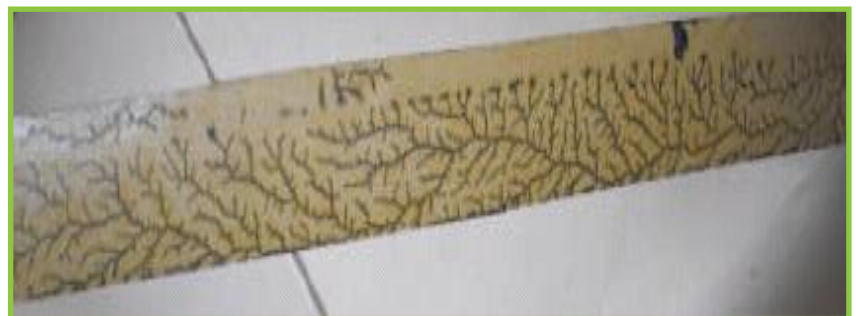
Tracking traces on paper insulation of a 150 kV cable
