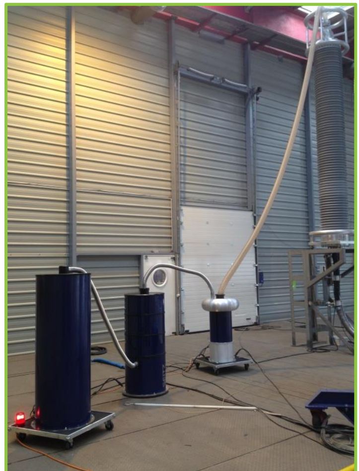
Damped AC test with PD measurements of a 320 kV HVDC cable
